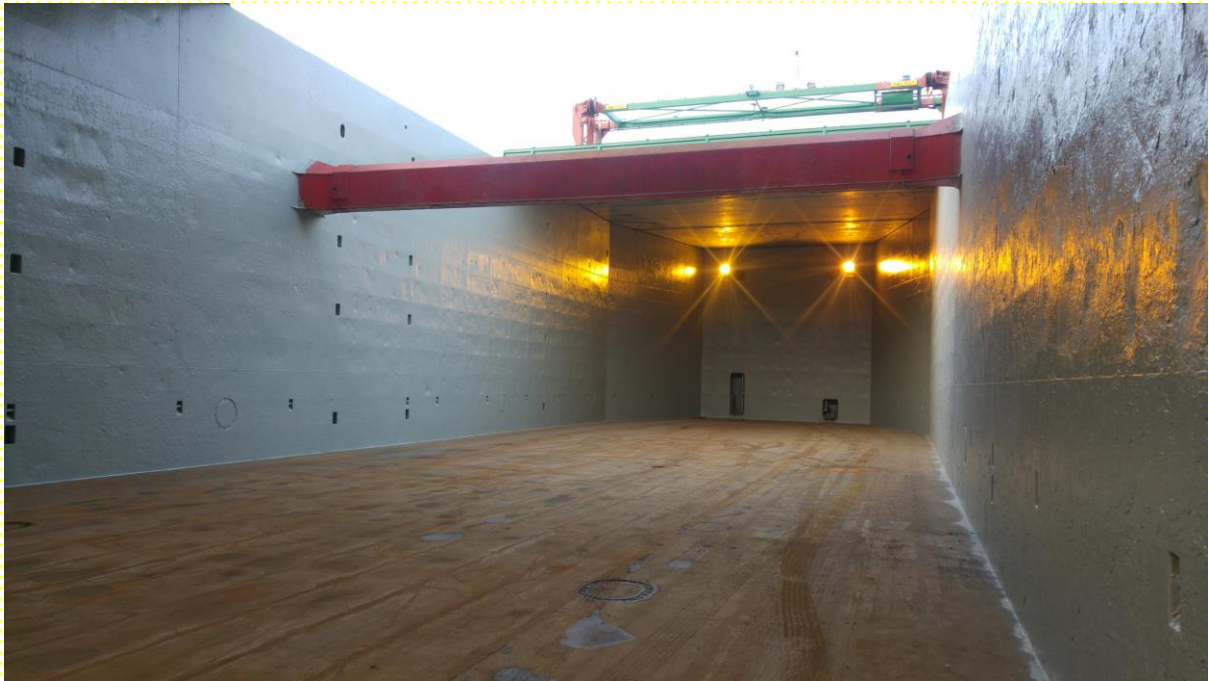
Hold (Forward) – Note Strong Beam Position
